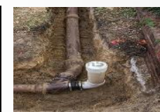
Trench for sewerage
