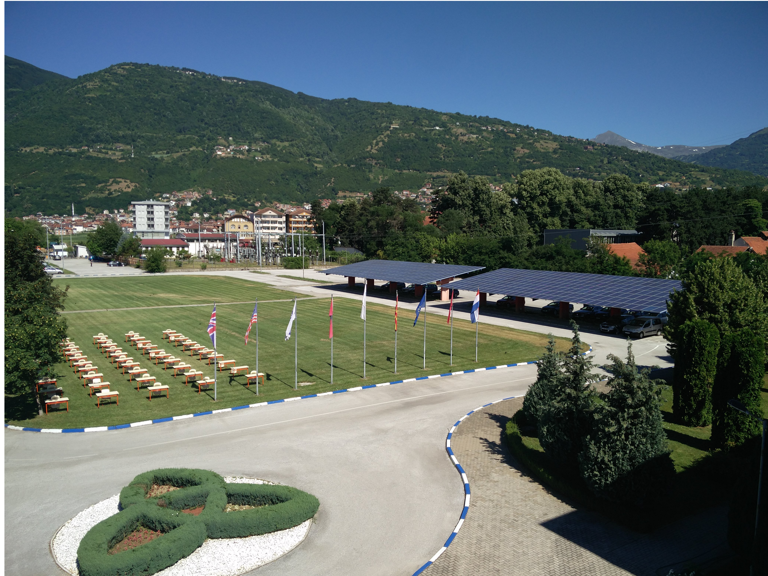
SEEU PV Plant 100kWp
